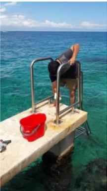
Adjusted angle of ladder for north pier for easier and safer use and repaired damages related to storm:
