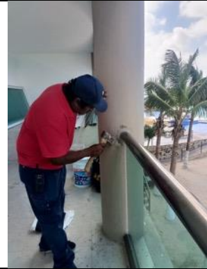
Repairs Cement Base in 9BN:
