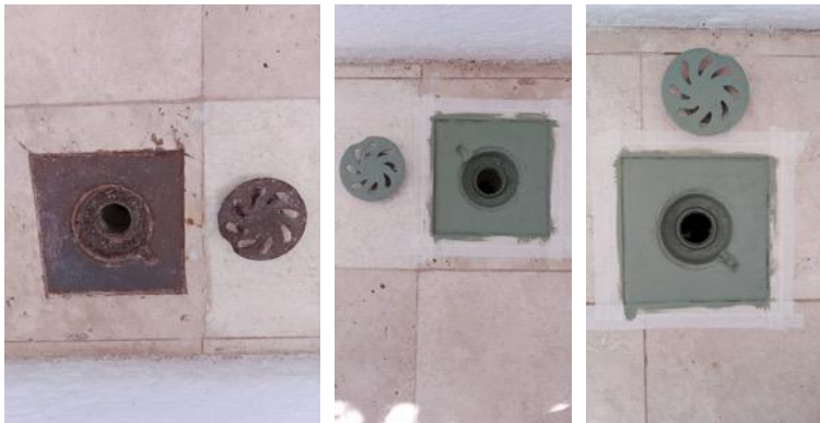
Repaired Leak into 9BN:
