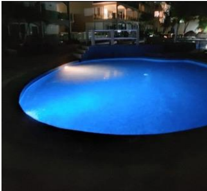
Pool Lights Replaced:
