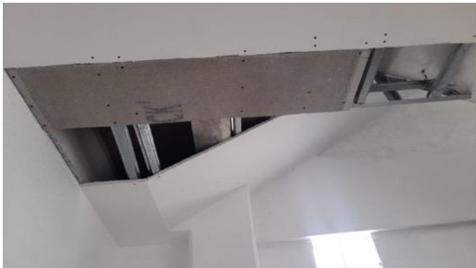
Pool Area Repairs:
