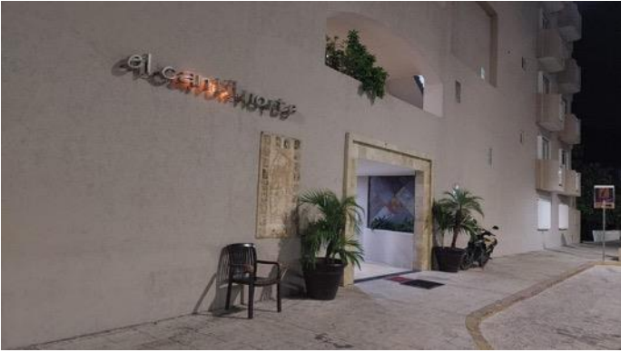
El Cantil North Sign Repaired:
