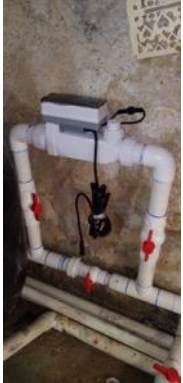
Installed new Chlorination Cell:
