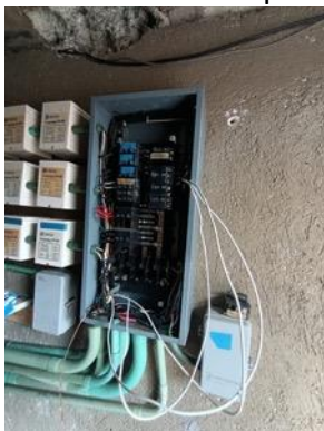
Installed Meter for Pool Water:
