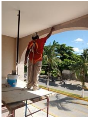
Massive Lamp – Cleaned, Removed Rust and Painted:
