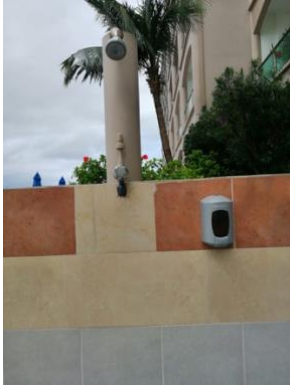
Bird Abatement Repairs:
