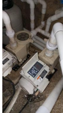
Pumps reinstalled and Pool System Cleaned and Restored: Bombas reinstaladas:
