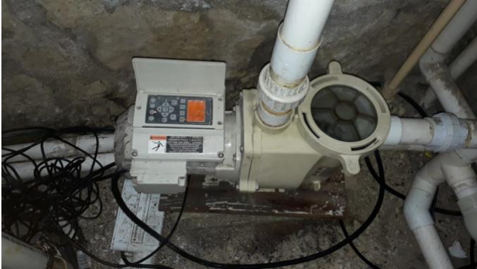
Pumps reinstalled and Pool System Cleaned and Restored: Bombas reinstaladas:
