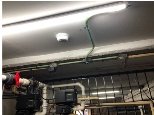
Installed Hazardous Gas (LP Gas) and Smoke Detectors Throughout the Complex:
