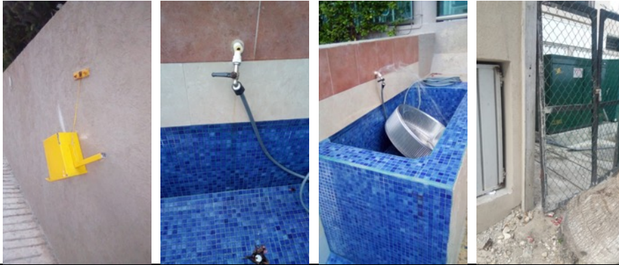
Serviced, cleaned and repaired AC balconies, nets and lids:
