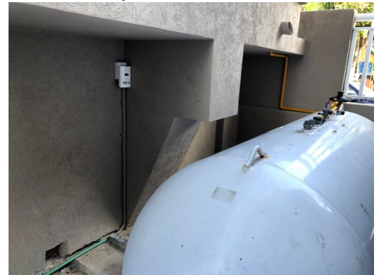
Installed Hazardous Gas (LP Gas) and Smoke Detectors Throughout the Complex:
