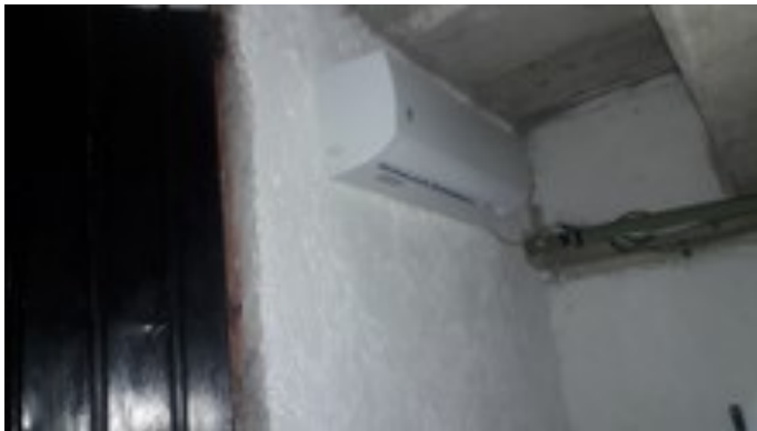
Installed drain lines in the cement:
