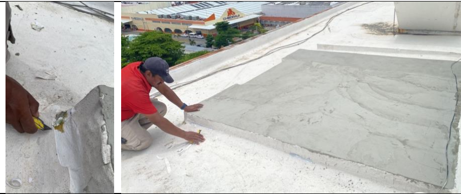
North Fence Repaired:
