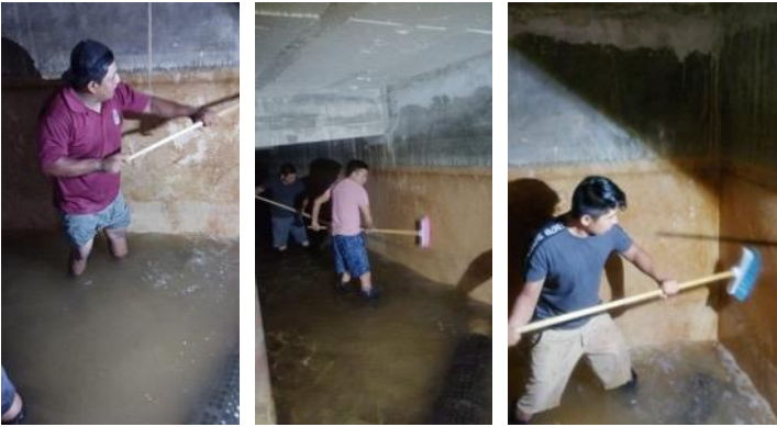
Cistern in South Tower Cleaned in the middle of the night:
