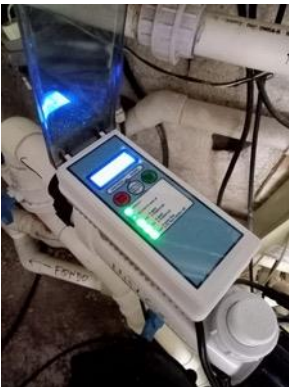
Installed new Chlorination Cell:
