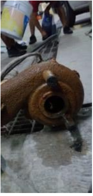
Repaired Sump Pump in North Garage:
