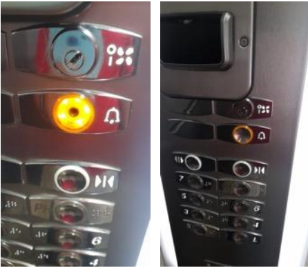
Elevator Button Repaired:
