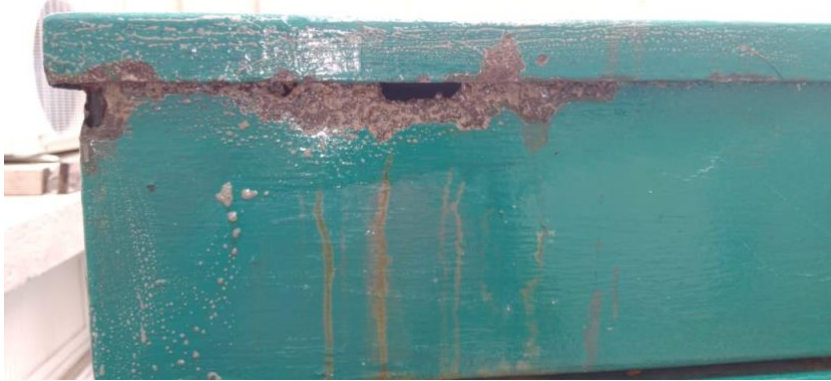
Transformer Rust Repair: -before/after-
