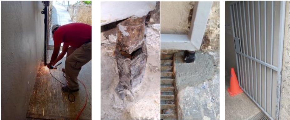
North Tower Raised Roof:
