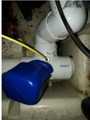
Replaced Temperature Sensor in Heat Pump – Heater for Hot Tub
