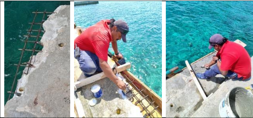
Pool Tile Repairs:
