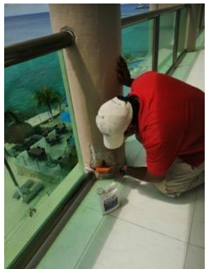
Column Rust and Cement Repairs:
