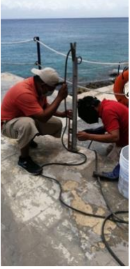
-Replaced Damaged Post-
