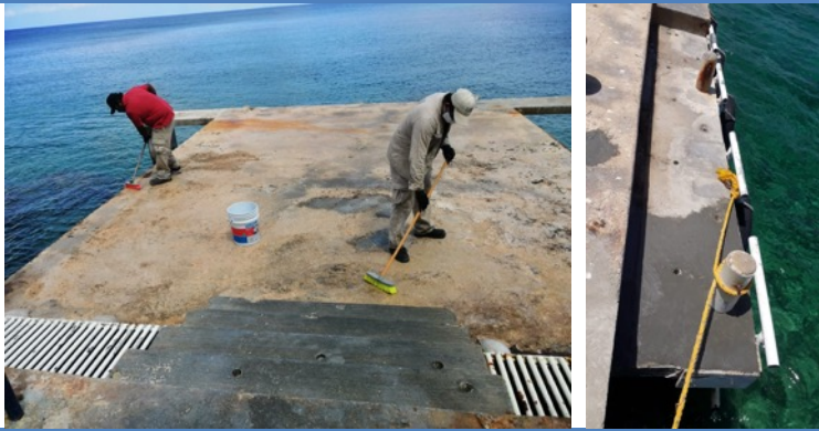
Repaired Lights for El Cantil Sign:
