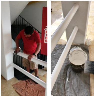
-Touched up Railings/Stairwells-
