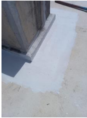
Cleaned Rooftops and Applied Sealer in Areas Needing Reinforcement:
