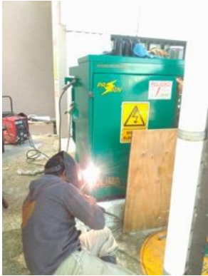
- Transformer Rust Repaired –
