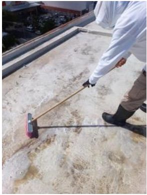
Cleaned Rooftops and Applied Sealer in Areas Needing Reinforcement:
