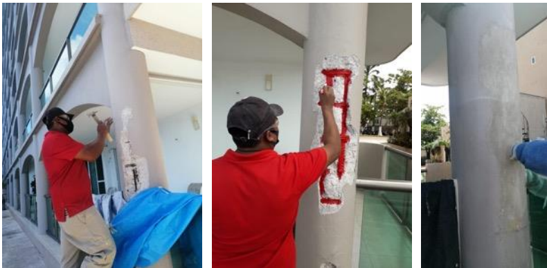
Rusted Rebar Repairs:
