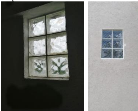
Repaired Bird Abatement:
