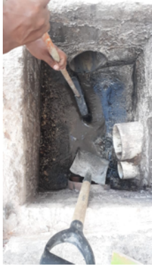
Cleaned Sewer Drain Registers:
