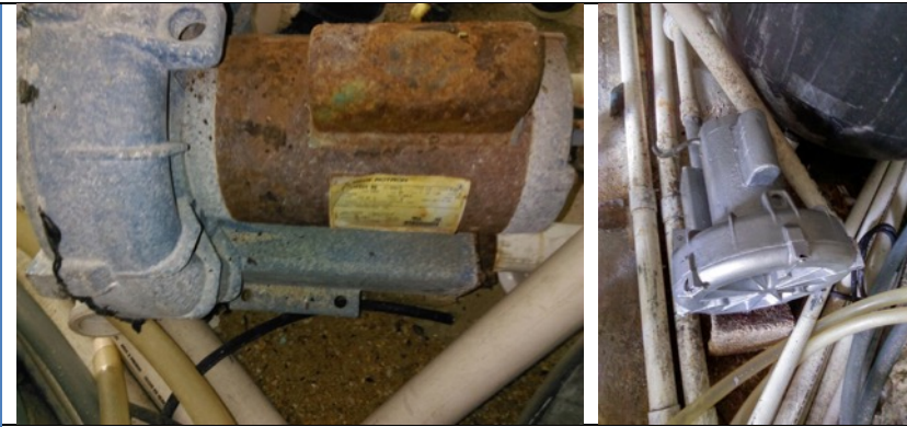
Grates that were broken, rusted and a danger to people were replaced:
