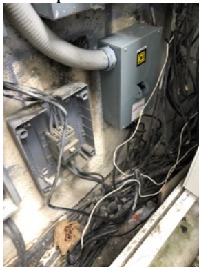
Example of Condo Electrical Installations in Poor Repair:
