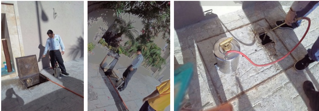
Hallway Drain's Covers Replaced:
