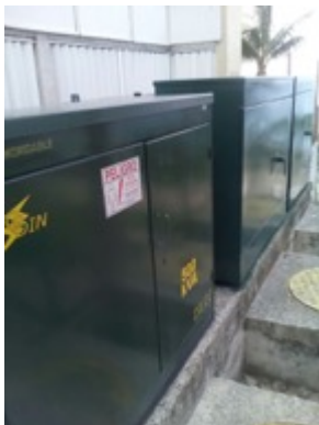
North Sign Repaired:
