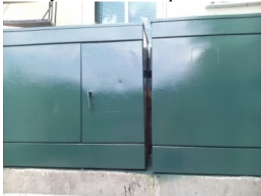
All transformers are now fully serviced and repainted:
