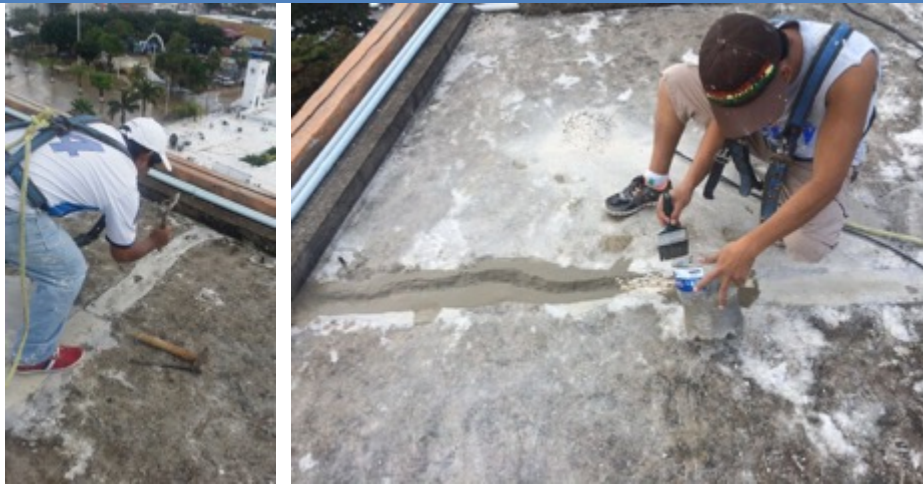
Picture of north tower roof now sealed:
